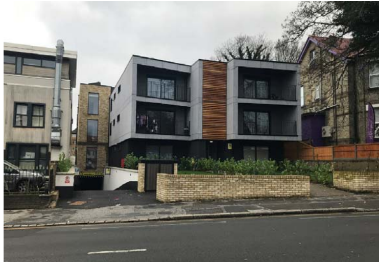
Figure 1 – front of site with adjoining premises
